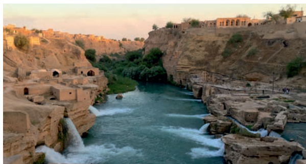
Water management in semi-arid regions 2,000 years ago: the Kārūn River in Shushtar (Khuzestan Province, Iran)
