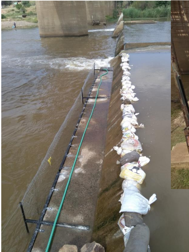
Protecting installation site against crocs, hippos and flooding
