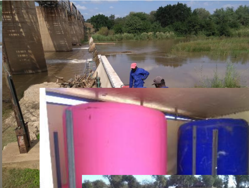
Installation of pumps at Oxford Weir
