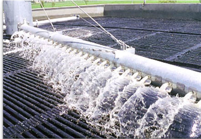
Sprinkler on top of a trickling filter filled with plastic media
