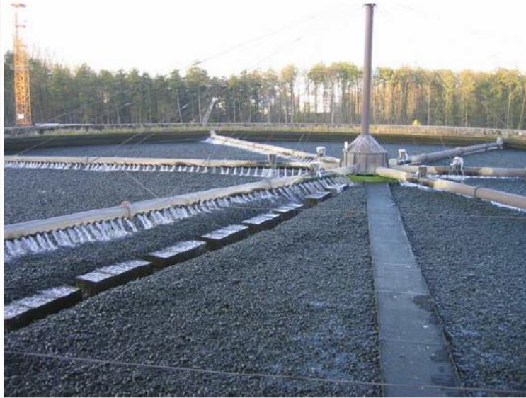
Topview of a trickling filter filled with lava rocks (Sindelfingen, Germany)
