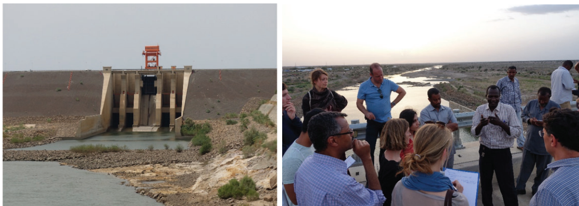
Picture 12. (Left) Upper Atbara Dam Complex in Sudan. (Right) Sudanese partners explain to the SaWaM team the operation of the Upper Atbara Dam Complex.
