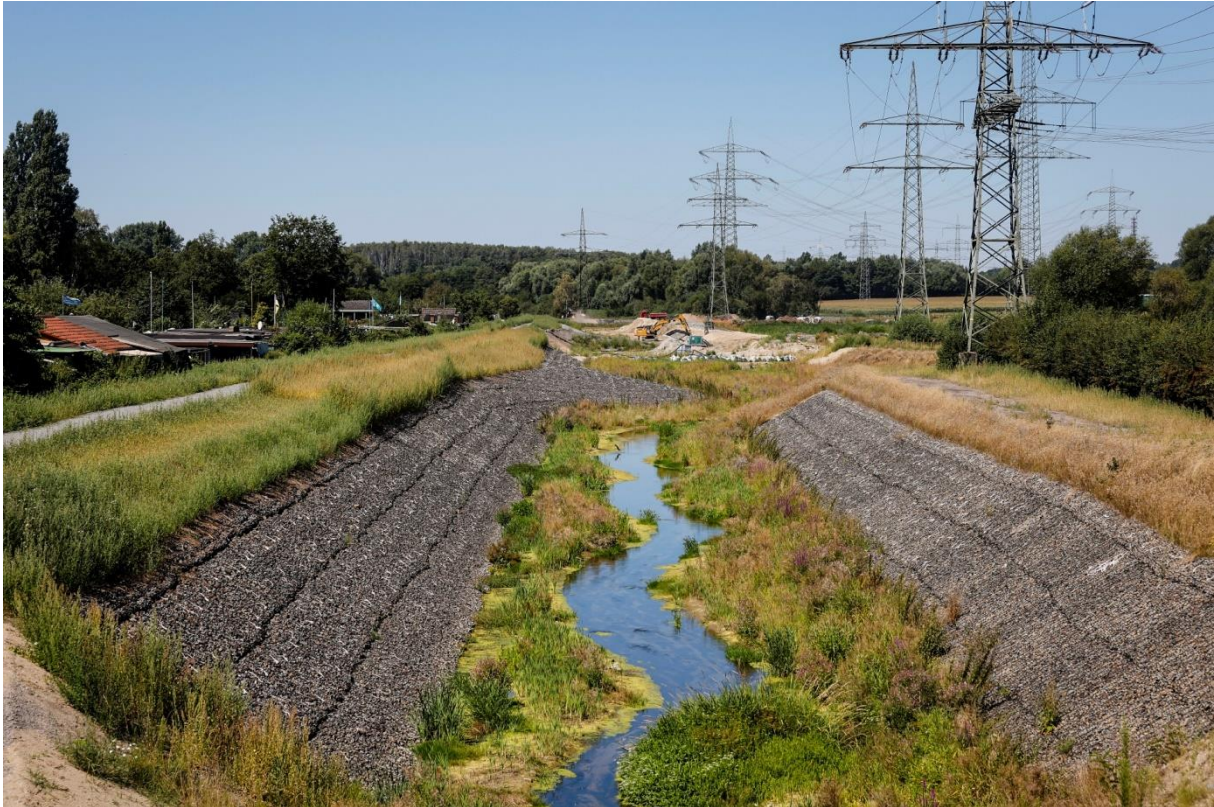
Figure 3: Restoration of a stream segment in the Emscher basin (photo: © Emschergenossenschaft, Rupert Oberhäuser).
